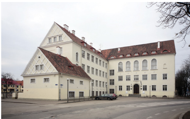
Figure 8. Pelgulinna Primary School in Tallinn (built – 1929).
