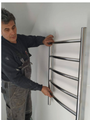
Figure 25. V. Bitenieks during improvement of a renovated house (2021).
