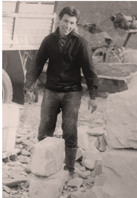
Figure 9. V. Bitenieks at the WEN construction site in Liepāja (1980).
