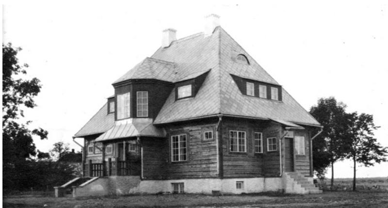
**Figure 10.** Veterinarian's house in *Raasiku* Parish built by the master builder Wassili Pander (?-?). The exterior cladding boards had not yet been installed (architect *K. Tarvas*; 1920s).
