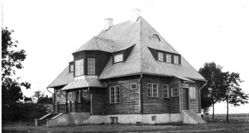
**Figure 10.** Veterinarian's house in *Raasiku* Parish built by the master builder Wassili Pander (?-?). The exterior cladding boards had not yet been installed (architect *K. Tarvas*; 1920s).
