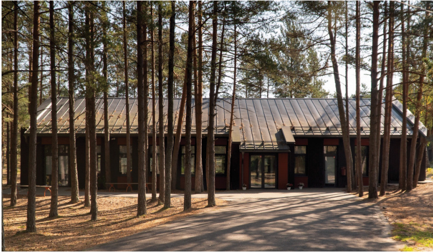
Figure 49. Old canteen building after reconstruction. Conference building (2014).
