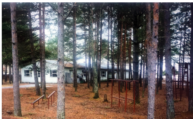
Figure 47. Old canteen building before reconstruction (2014).
