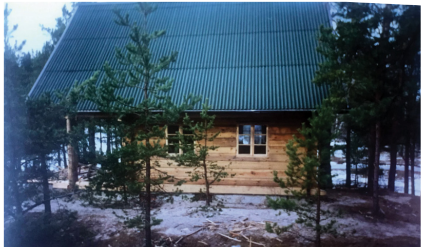
Figure 36. Facade of log house (1999).
