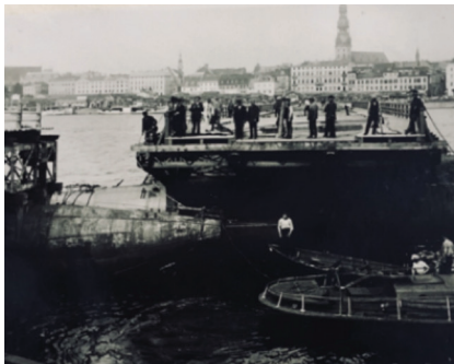
Figure 8. Construction of a Pontoon Bridge in Riga city (1931) [24].
