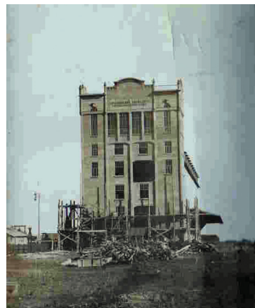
Figure 6. Construction of grain elevator in Altata (1916) [15].
