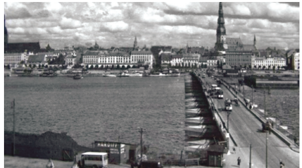
Figure 9. The Pontoon Bridge in Riga (in the 1930s) [25].
