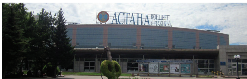
Figure 12. The main facade of the Palace of Tselinograd Virgin Land Developers (until March 2019 – Astana Concert Hall) (2017) [24].
