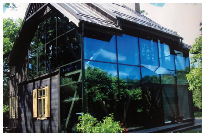
Figure 29. Residential building with garage at 5 Kanāla iela, Jūrmala city (2015) [50].
